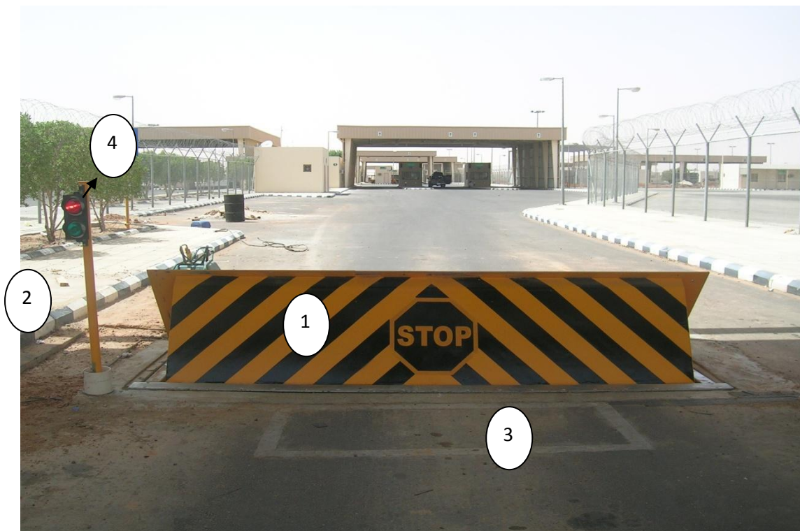
Picture 1. General View of Road blocker
